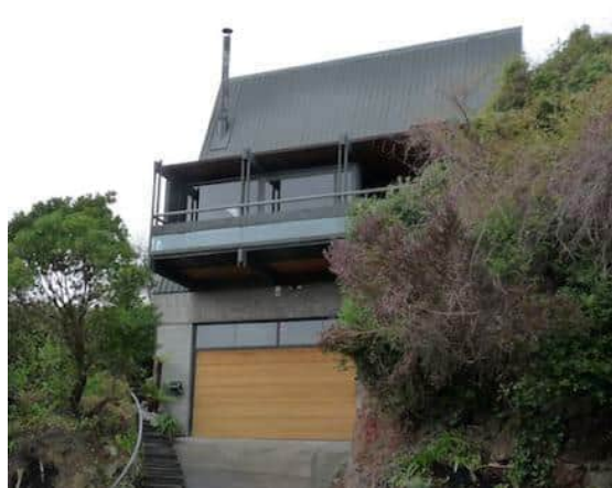
The former Hardie house.
